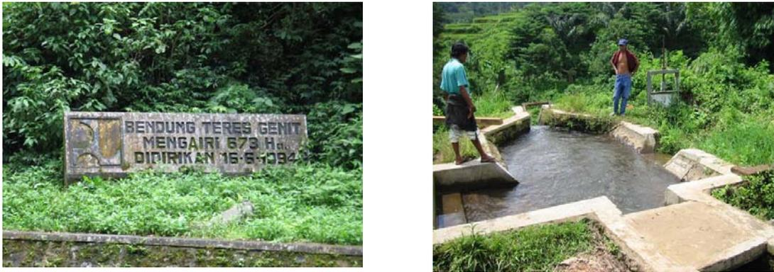
Figure 5.2 *Left: The previous MHP scheme was integrated into the Teres Genit irrigation system, which was constructed in 1994. Right: The majority of the civil structure was still in good condition and could be put back into operation for the MHP relatively easily*
